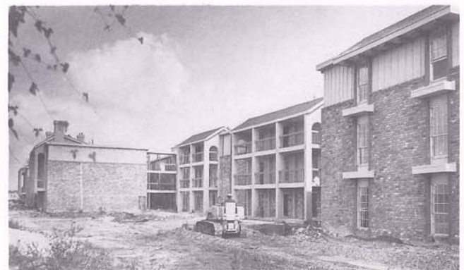
Apartment construction continues
