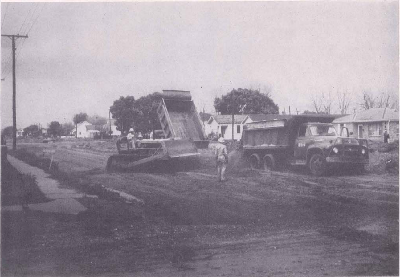
Working on the Franklin Avenue end of the section of the West Bank Expressway which will run from Franklin Avenue to Baratavia Boulevard and which is scheduled to be completed midsummer of 1956. This photograph was taken around the first of the year.
