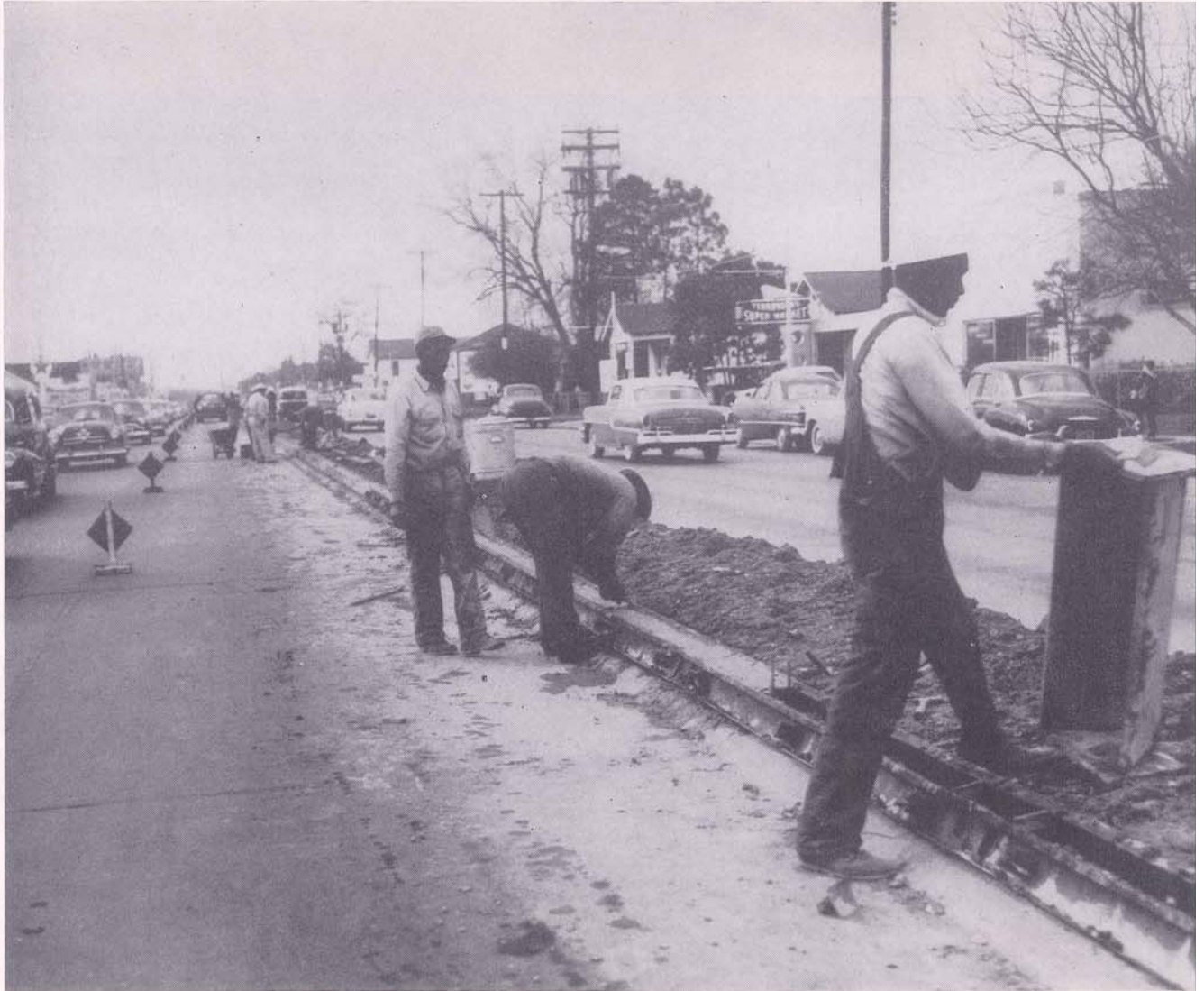
Working on the Airline Highway—widening and surfacing it from Shrewsbury Road (Severn) to Norco. This is part of its widening and covering with asphalt from Metairie to Spillway at a cost of $1,200,000—to be finished midsummer 1956.
