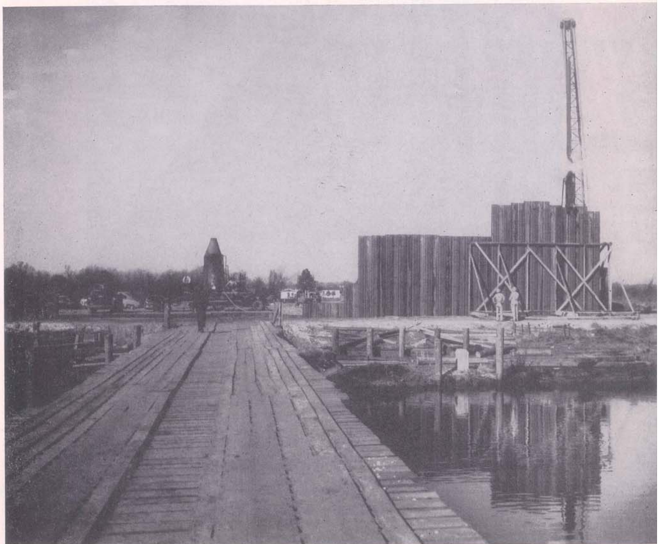
The preliminary work of driving pilings for the 6-lane concrete bridge over the 17th Street Canal in Metairie—part of the $1,150,000 Extension of Veterans Memorial Highway scheduled to be completed midsummer of 1956.
